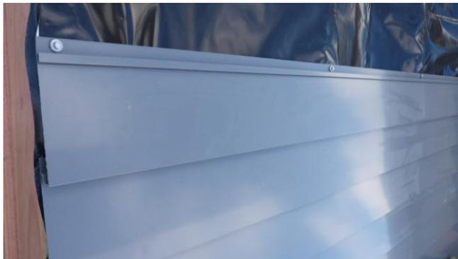
**Figure 2. General view of metal cladding and cladding fixing**
